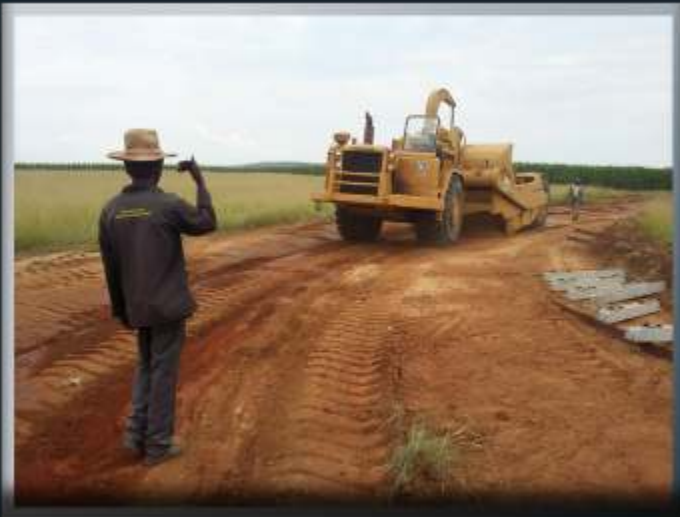
Below left: Easing the radius at the curve.
