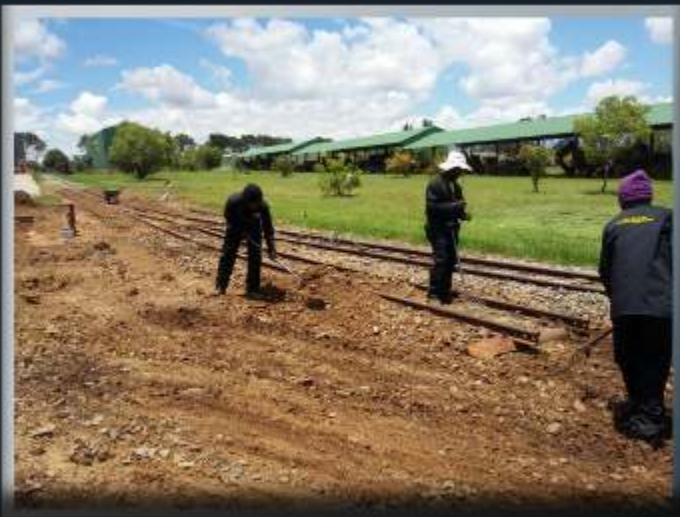
The line to the 150M shed was disconnected for a while to allow us to lay the curve and then we connected the 150M Shed storage line again.
