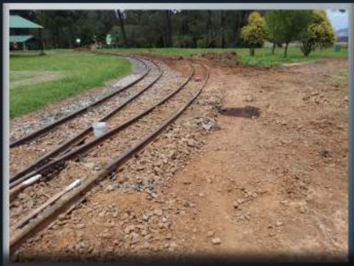
The line to the 150M shed was disconnected for a while to allow us to lay the curve and then we connected the 150M Shed storage line again.
