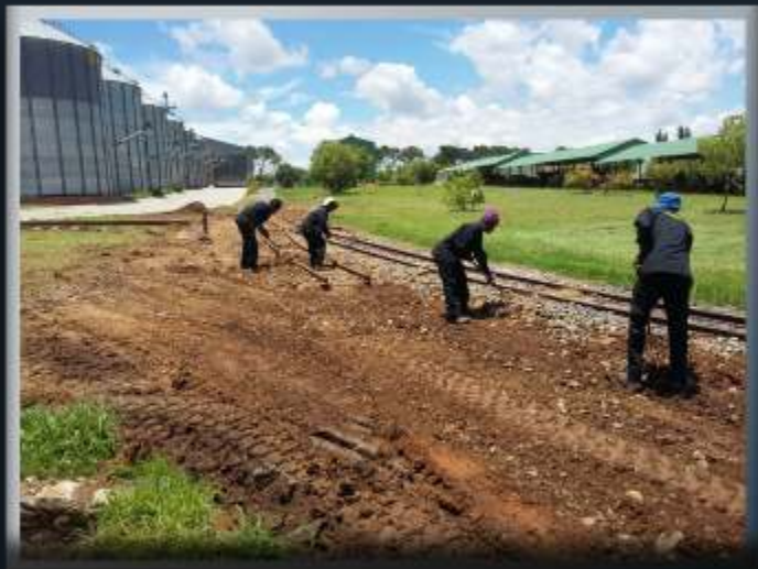
The line to the 150M shed was disconnected for a while to allow us to lay the curve and then we connected the 150M Shed storage line again.
