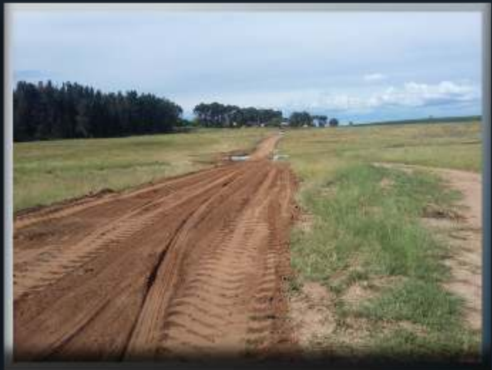
Below right: Filling up the ditch near the main culvert on the east side of the dam.
