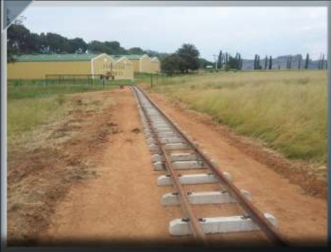
Below left: Easing the radius at the curve.
