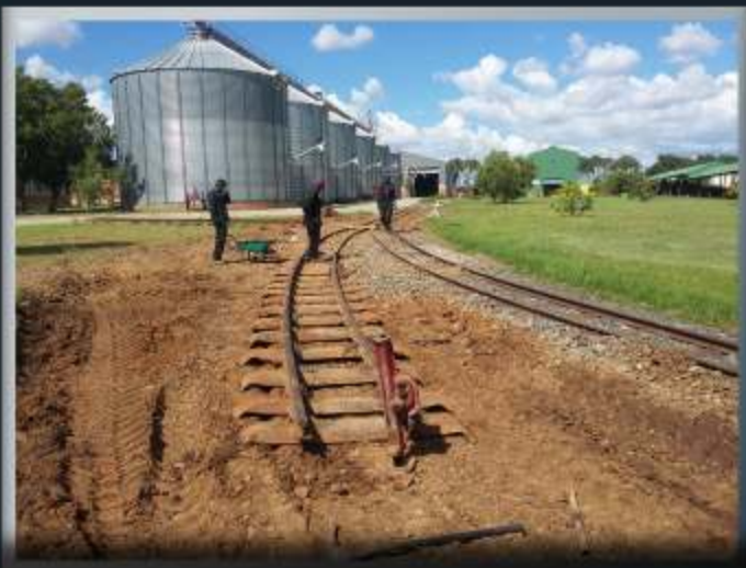
The line to the 150M shed was disconnected for a while to allow us to lay the curve and then we connected the 150M Shed storage line again.
