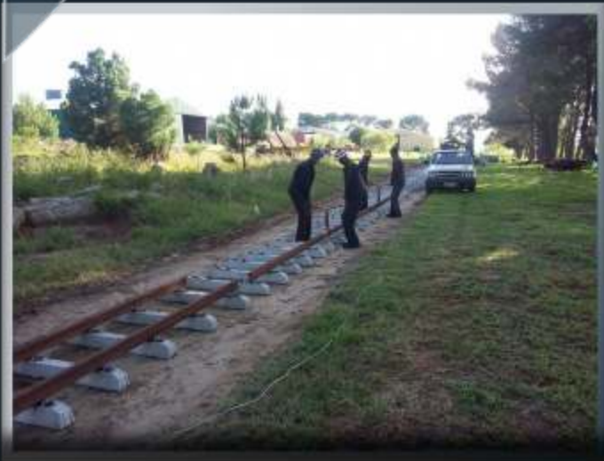
Below left: The straight to the 150M shed ballasted.
