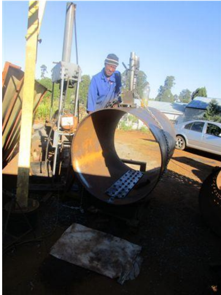
Fitting butt strap on front boiler barrel section
