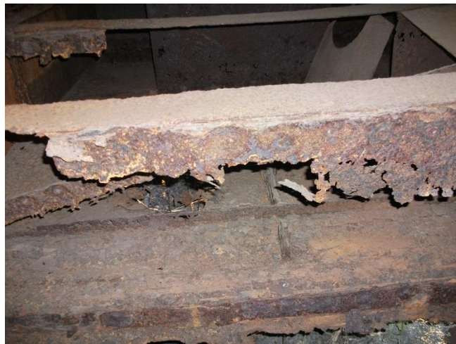
The wasted interior of the old tender tank.
