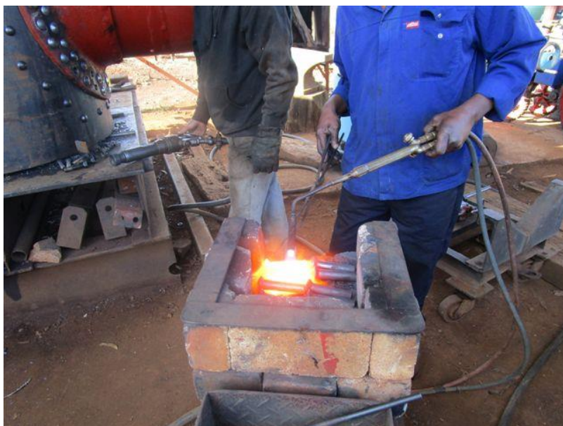
Heating up rivets
