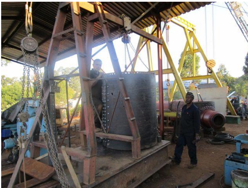
Putting the tube plate in position
