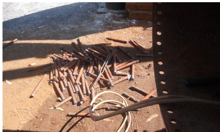
The crown stays after being cut off
