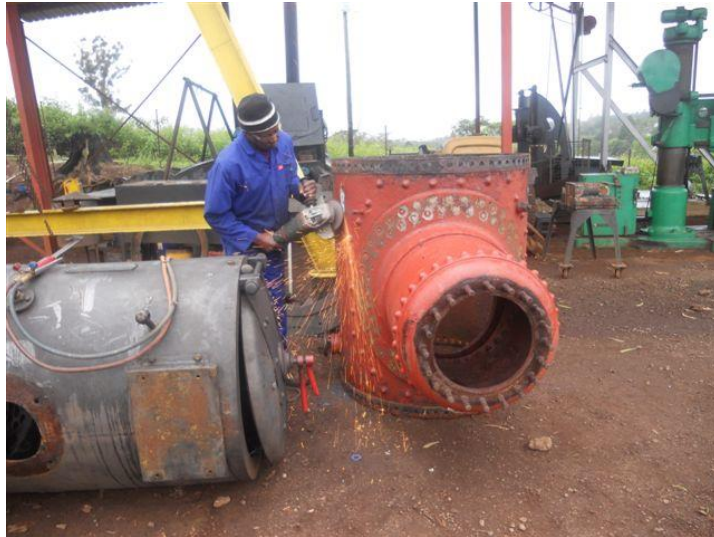
Stripping the dome section
