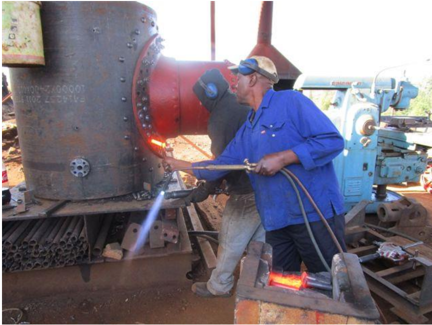
Riveting the dome
