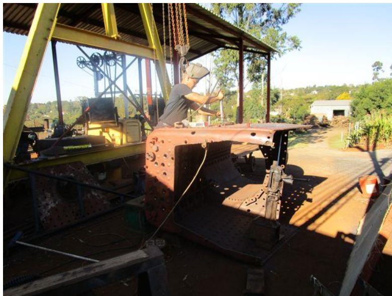
Scaling back end of boiler
