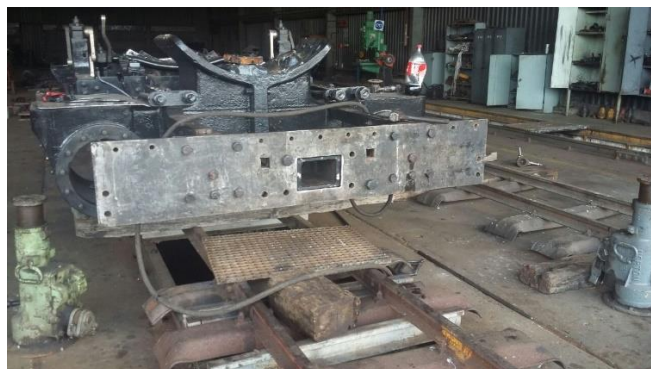
The repaired buffer beam
