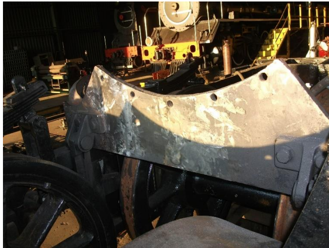
The boiler belly plate.
