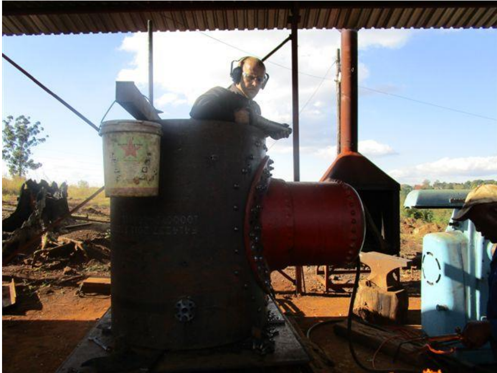
Riveting the dome to the boiler barrel
