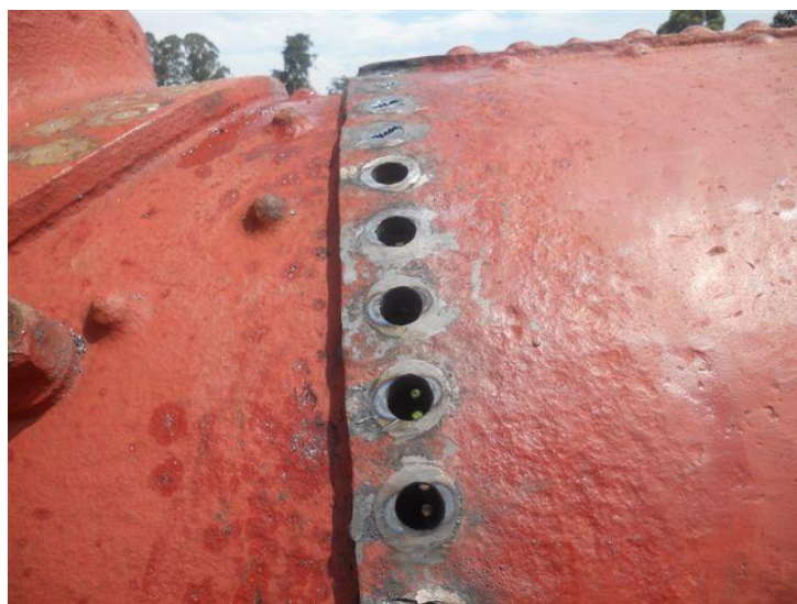
Rivets removed
