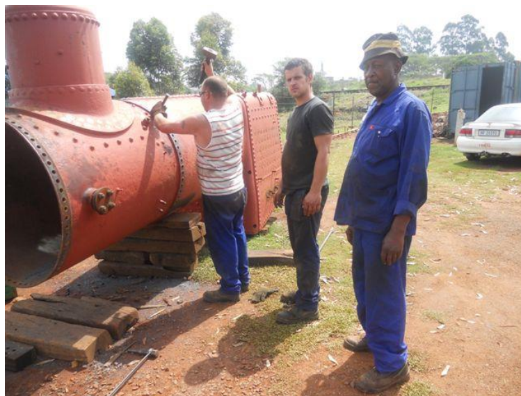
Removing rivets
